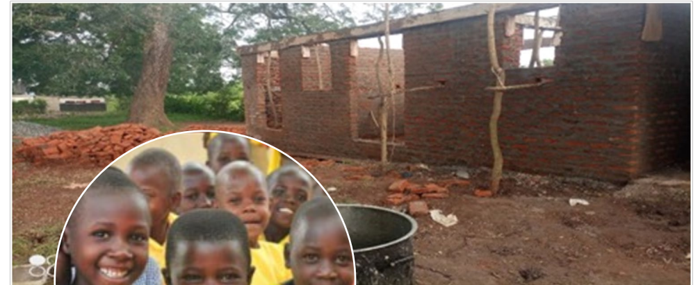
Above: Kitchen building work
